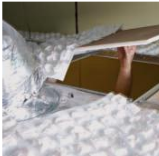
FIGURE 7 MACRO-ENCAPSULATED BioPCM INSTALLED IN TOP OF CEILING TILE IN A RETURN AIR PLENUM
