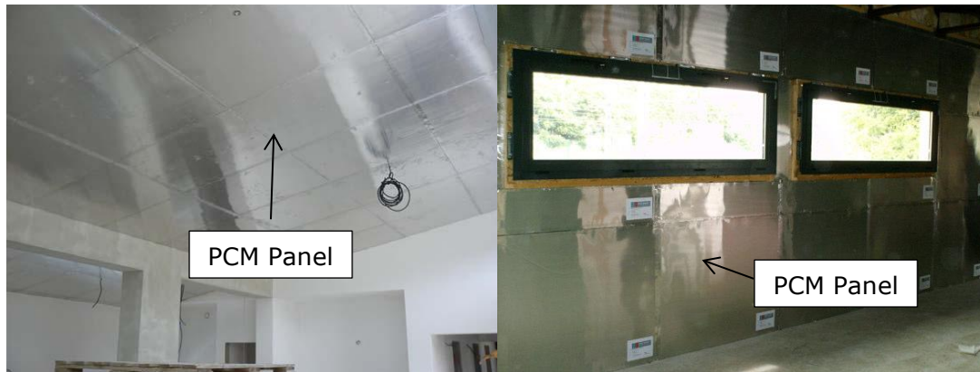
FIGURE 10. ENERGAIN PANELS ON THE INSIDE OF THE ROOF (LEFT) AND WALL (RIGHT). THE SURFACES WILL BE COVERED WITH WALLBOARD.
