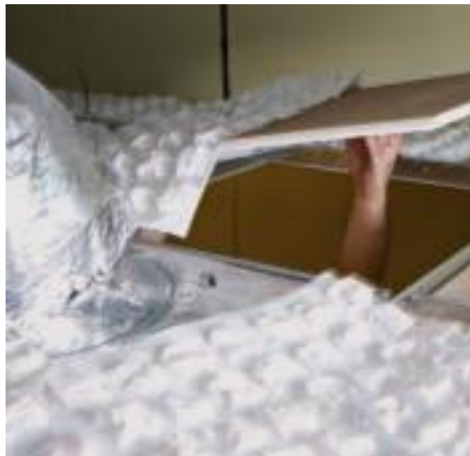
FIGURE 5. BioPCM INSTALLED ON TOP OF THE CEILING TILE IN A RETURN AIR PLENUM.
