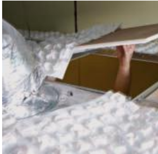
FIGURE 16 MACRO-ENCAPSULATED BioPCM INSTALLED IN TOP OF CEILING TILE IN A RETURN AIR PLENUM
