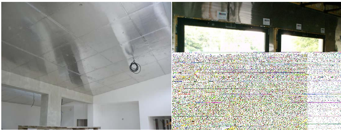
FIGURE 50. ENERGAIN PANELS ON THE INSIDE OF THE ROOF AND WALL. THE SURFACES WILL BE COVERED WITH DRYWALL.
