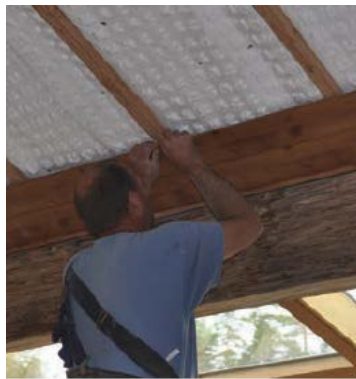
FIGURE 2: PHASE CHANGE ENERGY SOLUTIONS' MARKETING MATERIAL: PCM INSTALLED WITHIN WOOD FRAMED ROOF
