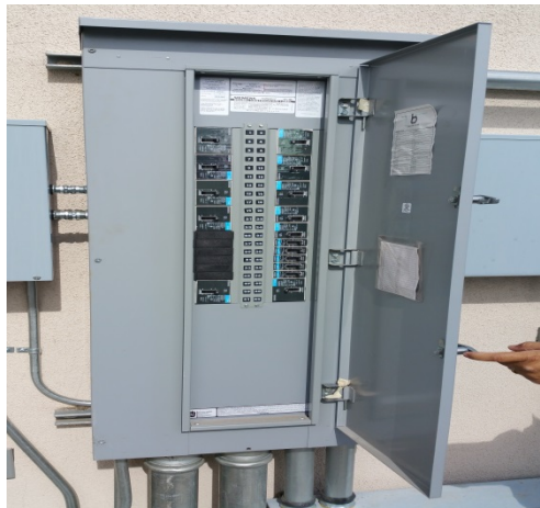
FIGURE 10: TRAINING FACILITY'S BUILDING METERING SYSTEM ON THE TWO ELECTRICAL PANELS
